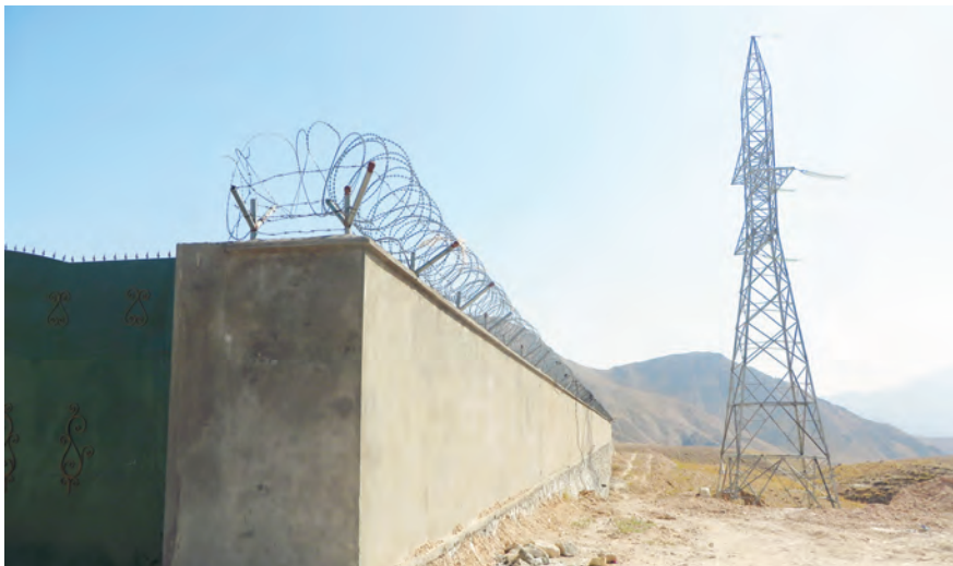
A Northeast Power System terminal tower ending without connection to the Nejrab District substation. (SIGAR photo)
