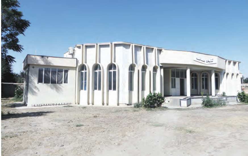
The Kunduz library constructed with funds from the Good Performers Initiative, Kunduz Province. (SIGAR photo)
