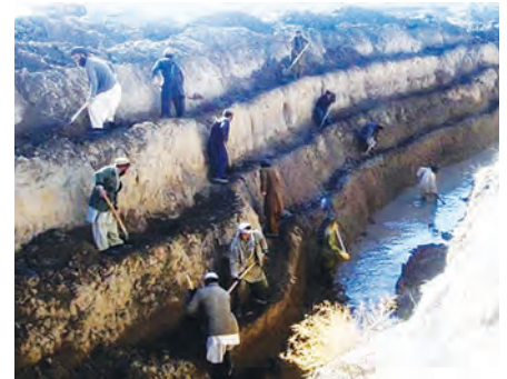
Villagers working under a USAID grant terrace and clear an irrigation canal in Logar Province, 2013. (USAID photo by Ahmad Salarzai)
