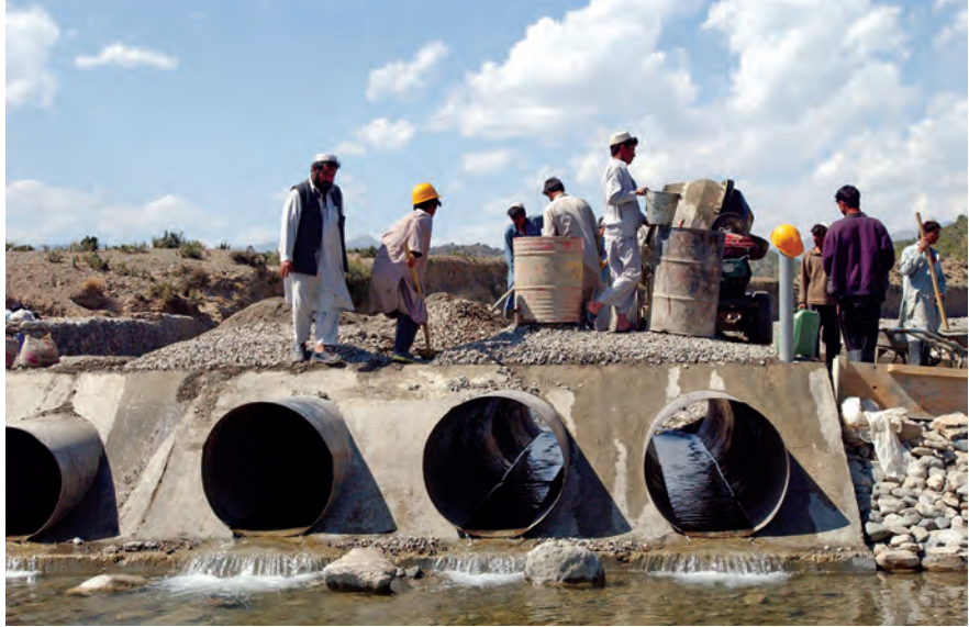
Afghans work on a CERP-funded aqueduct system in Khost Province, 2006. (DOD photo by Staff Sgt. Robert R. Ramon)
